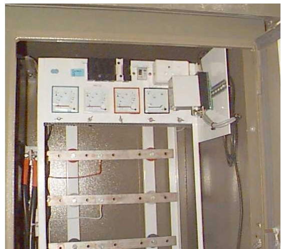
Below right: Desta type Mini-sub LV chamber (Note: the SLP on the right, is a little larger than a conventional amp meter)
